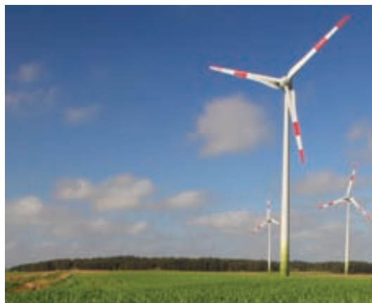
Assets range from renewable energy to hospitals, each with distinct risks
